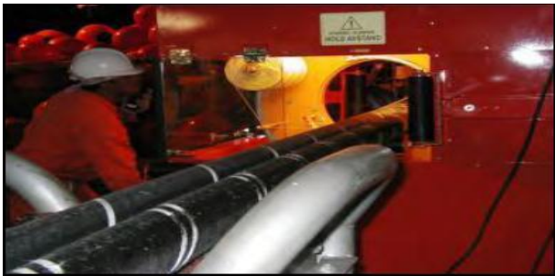
Fig.1 Bundling power cable for laying [1]
